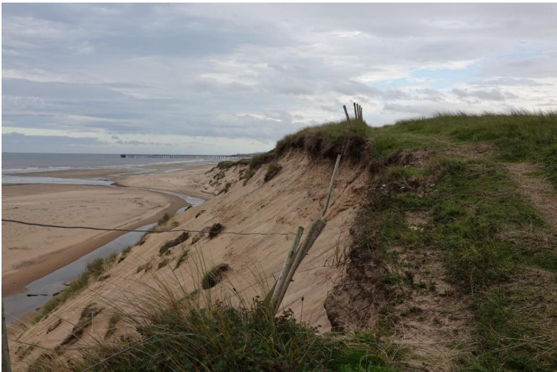
Figure 3.7 Sand fence on crest of dune now on dune face adjacent to golf course
